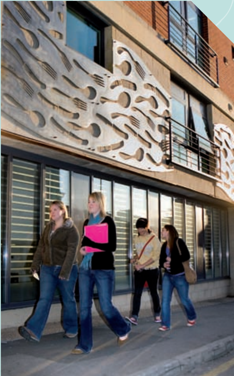
Accommodation at Exchange Works
