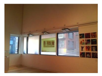
Six windows in two rows of three, visible from the street. Each one measures approx 1.75m \* 1.75m. Double glazed with the interior glass laminated with BLINK film. When switched on the film is transparent. When switched off the window is frosted. Above each window is a projector set up to project an image onto the frosted glass to be viewed from outside the gallery in the street. Images are more visible on darker days or during the evenings.
