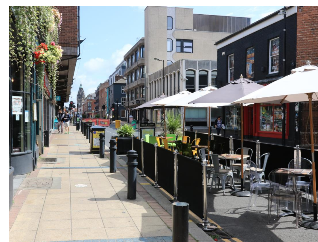
Division Street Pedestrianisation, Sheffield
