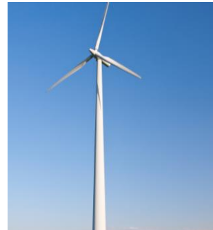
Horizontal Axis Wind Turbine
